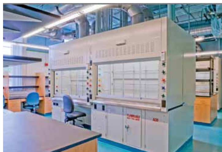
▲ VAV fume hoods - organic laboratory - Pearson Michael Chemistry Building, Tufts University. Goldman Reindorf Architects, Inc.
