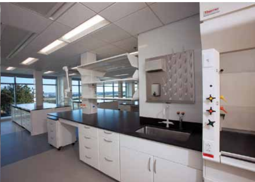
▲ Fume hood alcove to the right with chilled beams in upper left. PHOTO COURTESY OF LEE BRAUER.
