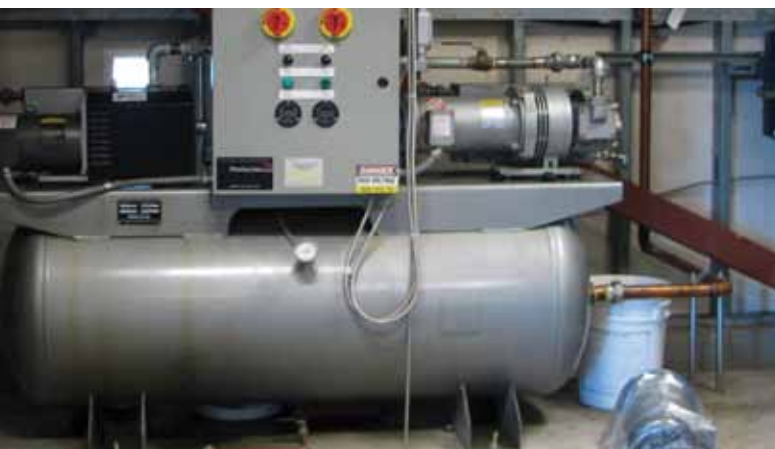
▲ A common configuration for a small central vacuum pumping system: two pumps and a control panel mounted on a ballast tank in the basement.
