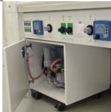
◀ With local vacuum pumping systems, the pump fits under a fume hood, with manual or electronic vacuum controls mounted on the fume hood panels.
