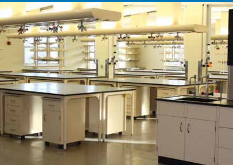
▲ Custom overhead service carriers, mobile cabinets, and fixed steel casework. Project: Carnegie Mellon University, Pittsburgh, PA.
